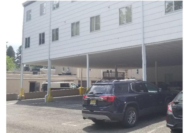
Pervious pavement can be installed in the back parking lot to capture, treat, and infiltrate parking lot runoff. Downspout planter boxes can be installed at the bases of the downspouts connected to the support beams at the southeast corner of the building to capture and filter stormwater. A preliminary soil assessment suggests that more soil testing would be required before determining the soil's suitability for green infrastructure.
